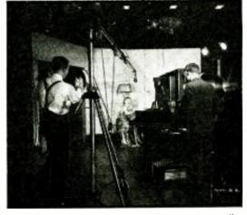
Left—the Television Traffic Man, watching the action in the studio, monitors the program on the Kinescope above the window. A breast microphone connects directly with . . . . Right—the Iconoscope Camera Man, who is here shown putting Miss Hildegarde "on the air" via NBC-RCA at Radio City.
